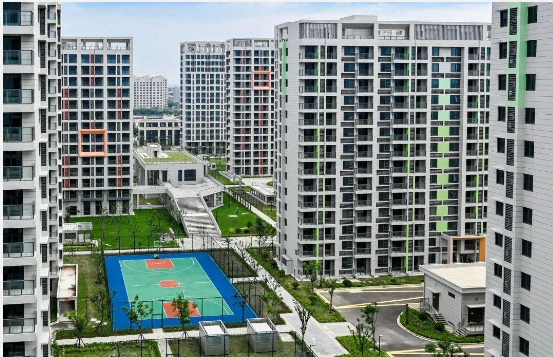
Figure 35 On-site photo of "Fengfa Future • Lingang Community"
