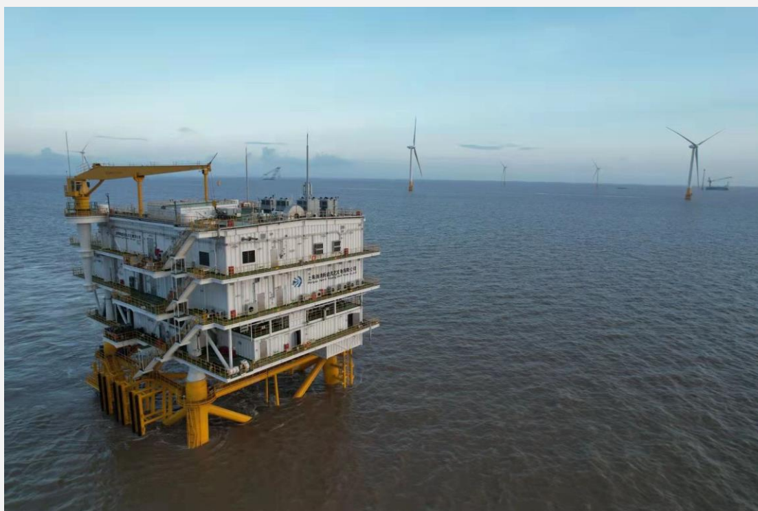
Figure 14 Offshore Booster Station of the Fengxian Offshore Wind Proposal
